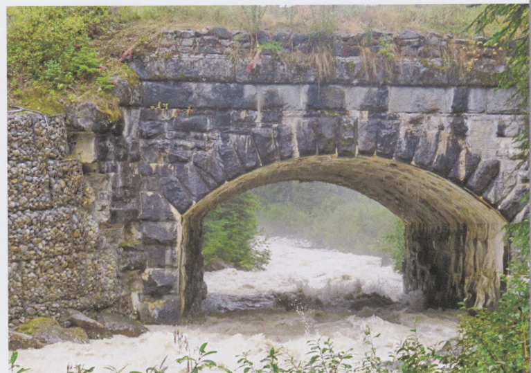
Original Rail Bridge over the Illecillewaet River
